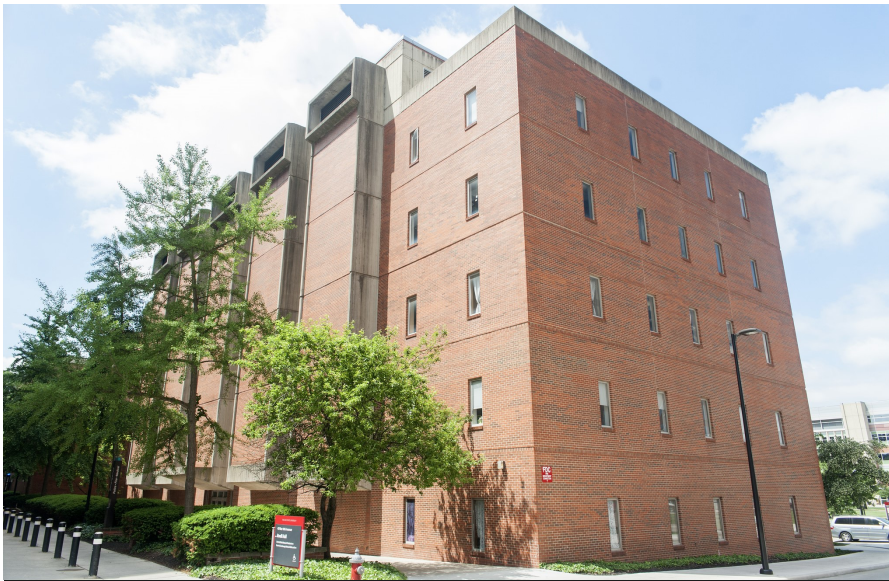
Atwell Hall, School of Health and Rehabilitation Sciences
